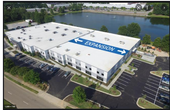
Figure 10: is a picture of the ELOS MedTech building expansion proposal in Nashville Tennessee. This company has been making implant products Nobel Biocare for over 25 years. Both Nobel and ELOS know the manufacturing tolerances of their products.
